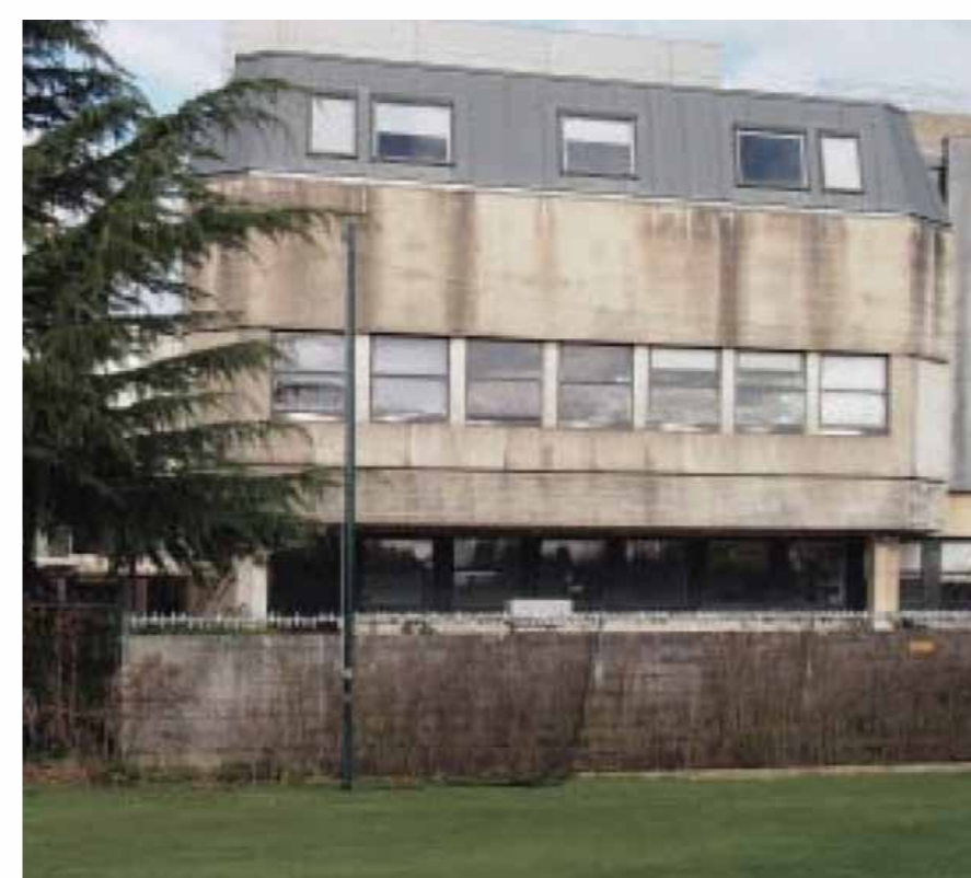
Existing facade current condition
