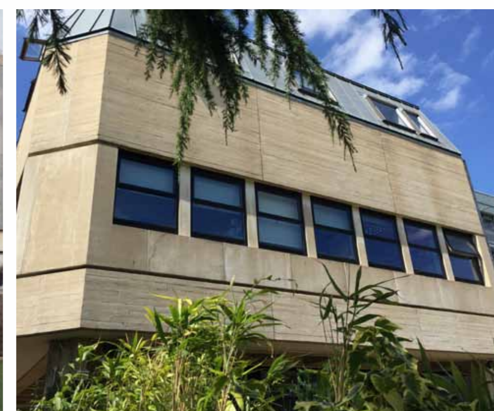
Existing facade after cleaning
