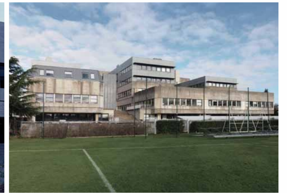
Photograph of the building in its current condition
