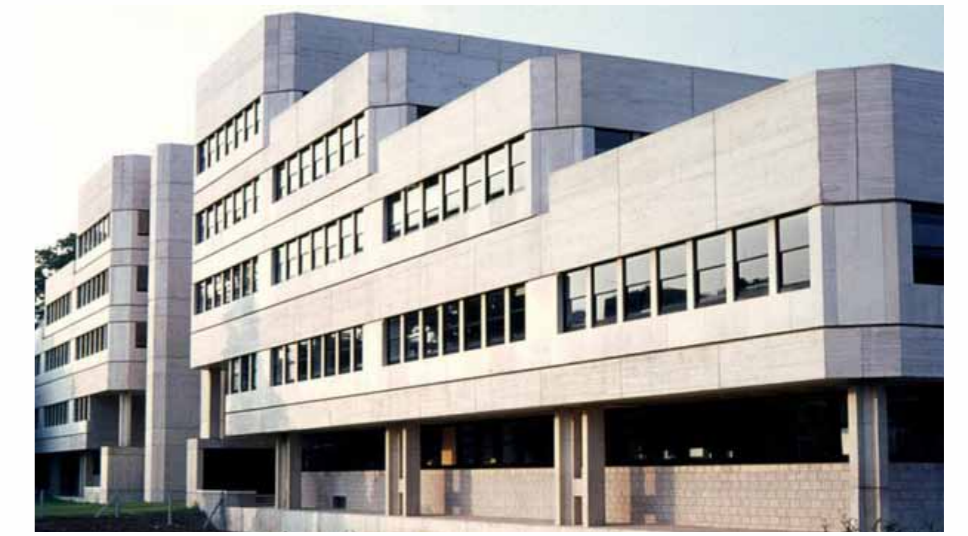
Photograph of the original building in 1970
