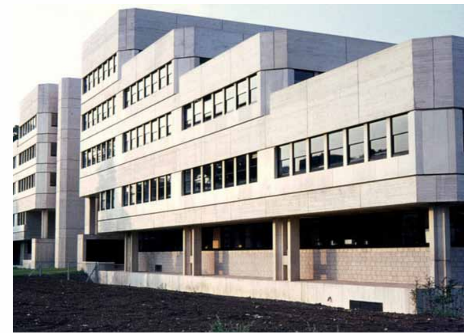
Photograph of the original building in 1970
